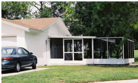
Unacceptable: prefabricated screen room.
