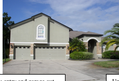
Unacceptable: entry and garage out of proportion to rest of house
